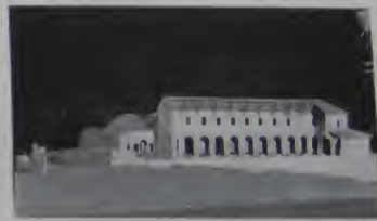
Fig. 5c. S. Sebastiano. Section of building, exterior, facing south.
